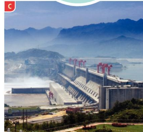
▲ The Three Gorges dam on the Yangtze, over 600 km from Chongqing. Ships pass it using locks. There's also a special lift for ships – the biggest lift in the world.
