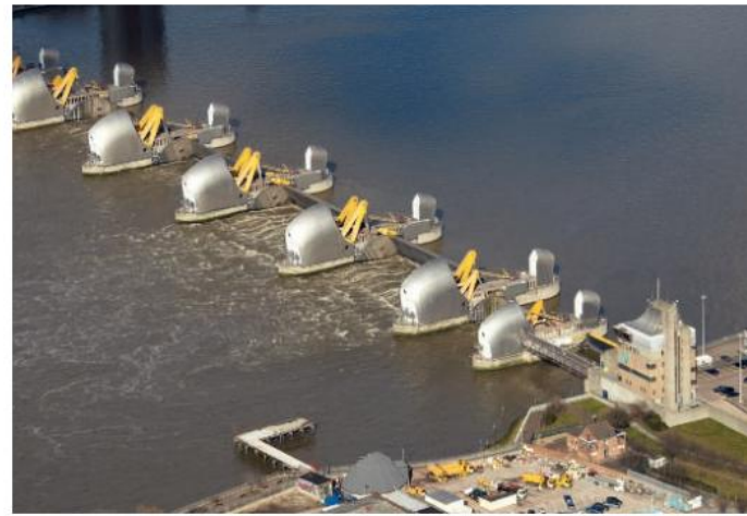
▲ The Thames Barrier, closed. It's always closed during a storm surge in the North Sea, to protect London.
