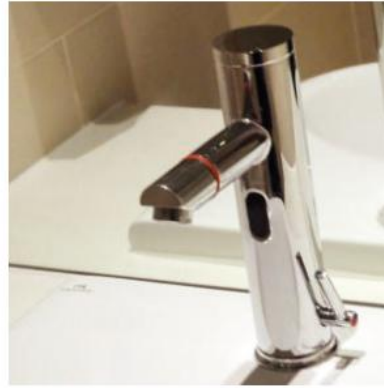
▲ There are no taps or light switches. Sensors detect when you want to use water, or enter a dark room.
