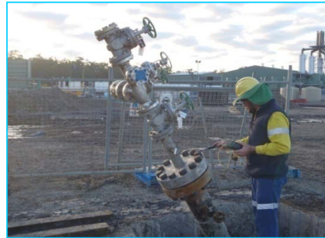
Panel 2 - injection well head
