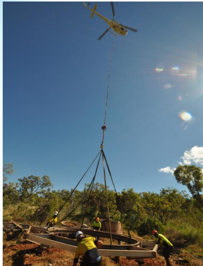
Right: Universal Drilling Platform being lowered onto drill location
