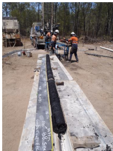
Coring by twinning open PCD hole ML002 a partial section of the B8 seam is shown
