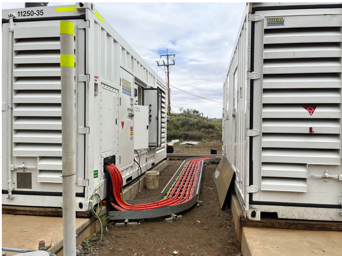
Image 1 – Generators installed at the GAM Plant site, with high voltage cables installed.
