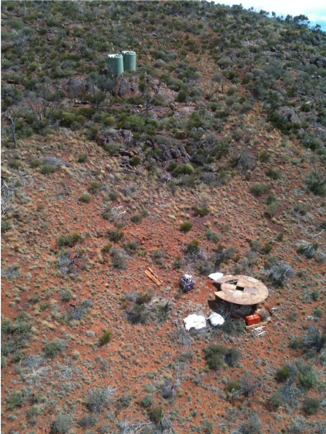
Figure 2 – Drill platform partly constructed on a 20 degree slope
