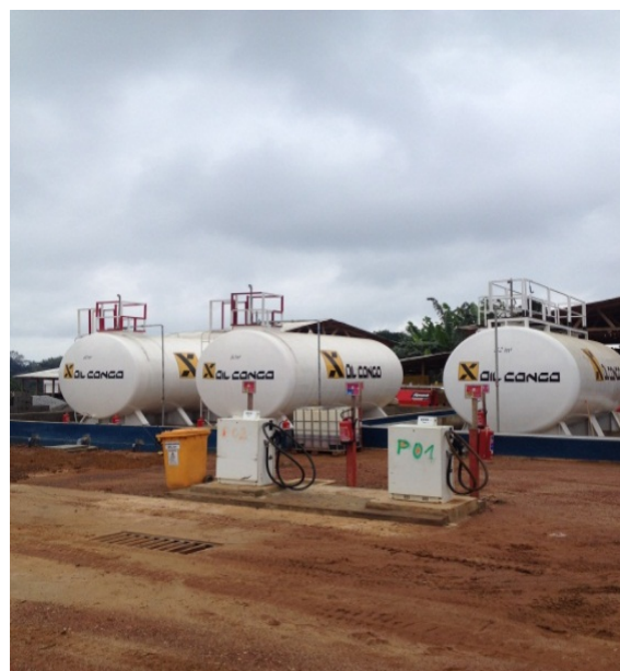
Figure 6: 50,000 Litre Fuel Storage Tanks at Mayoko
