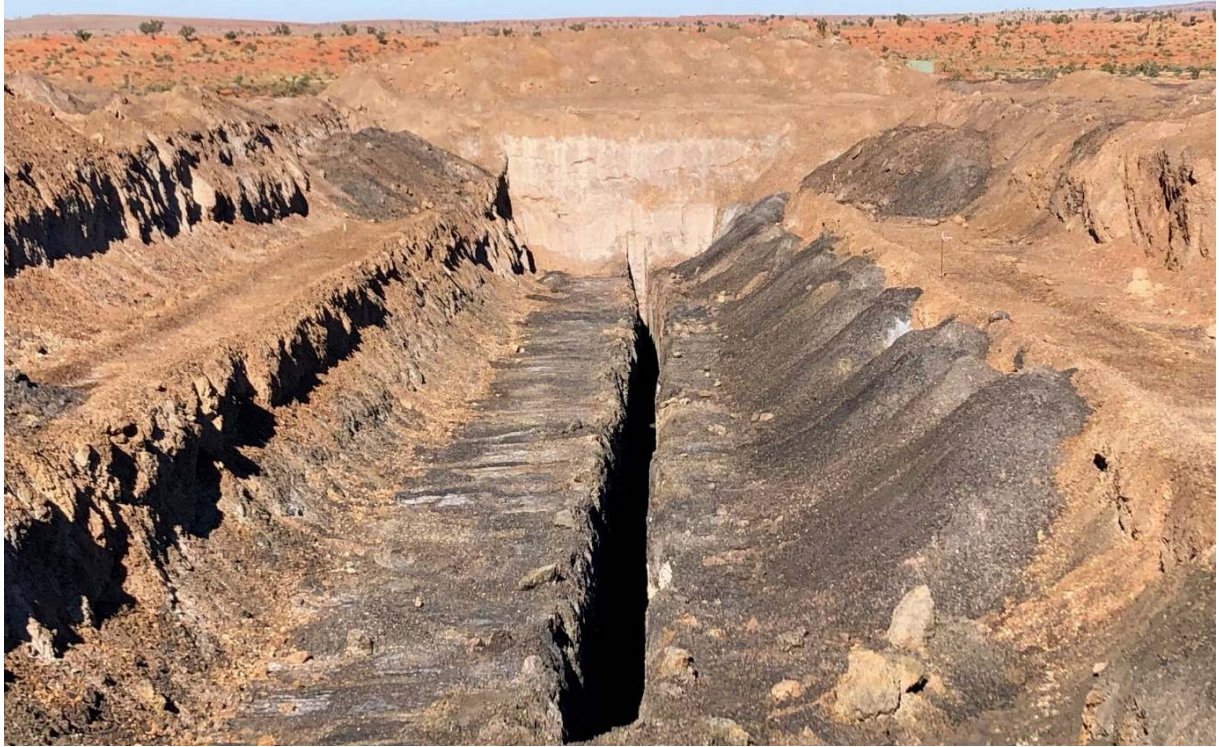
Figure 5: Trenching of the heap leach at the Nifty Copper Project
