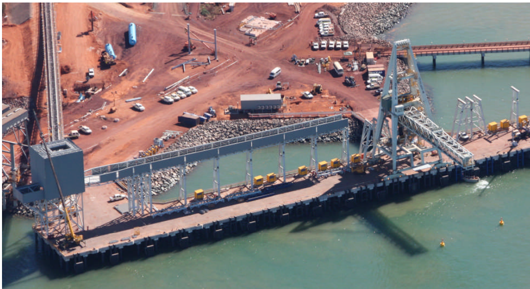
Utah Point multi user berth, with locally constructed, Delta 7,500 Tonnes/hour ship loader
